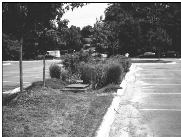
Figure 2: Parking Lot Island Turned Bioretention
