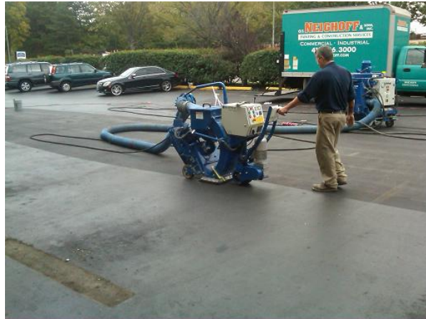
Figure 9 Coal Tar Remediation Site
