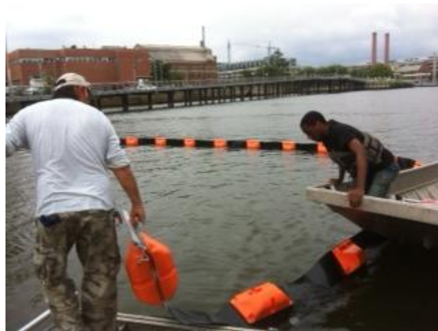
Figure 11 Installation of Booms Around ECC Dock in Southwest DC
