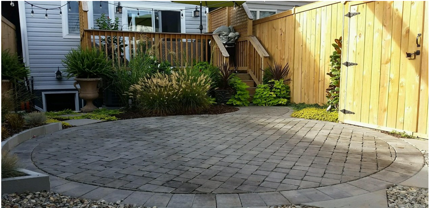
RiverSmart Permeable Paver Project
