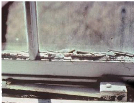
Paint-based lead hazards in the home can look like this....
