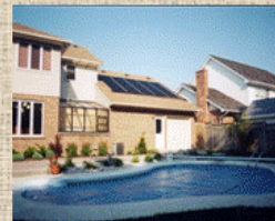
Roof-mounted solar pool heating system
