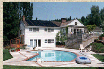
Roof-mounted solar pool heating system
