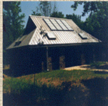
Campground solar hot water system
