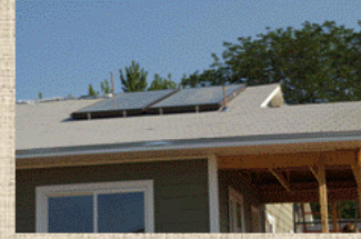
Habitat for Humanity house with solar collectors
