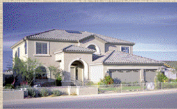
Residential solar hot water system
