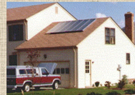
Solar water heating
