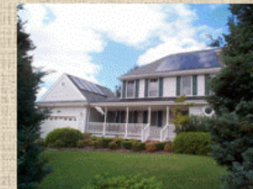
Chesapeake VA home with solar heating
