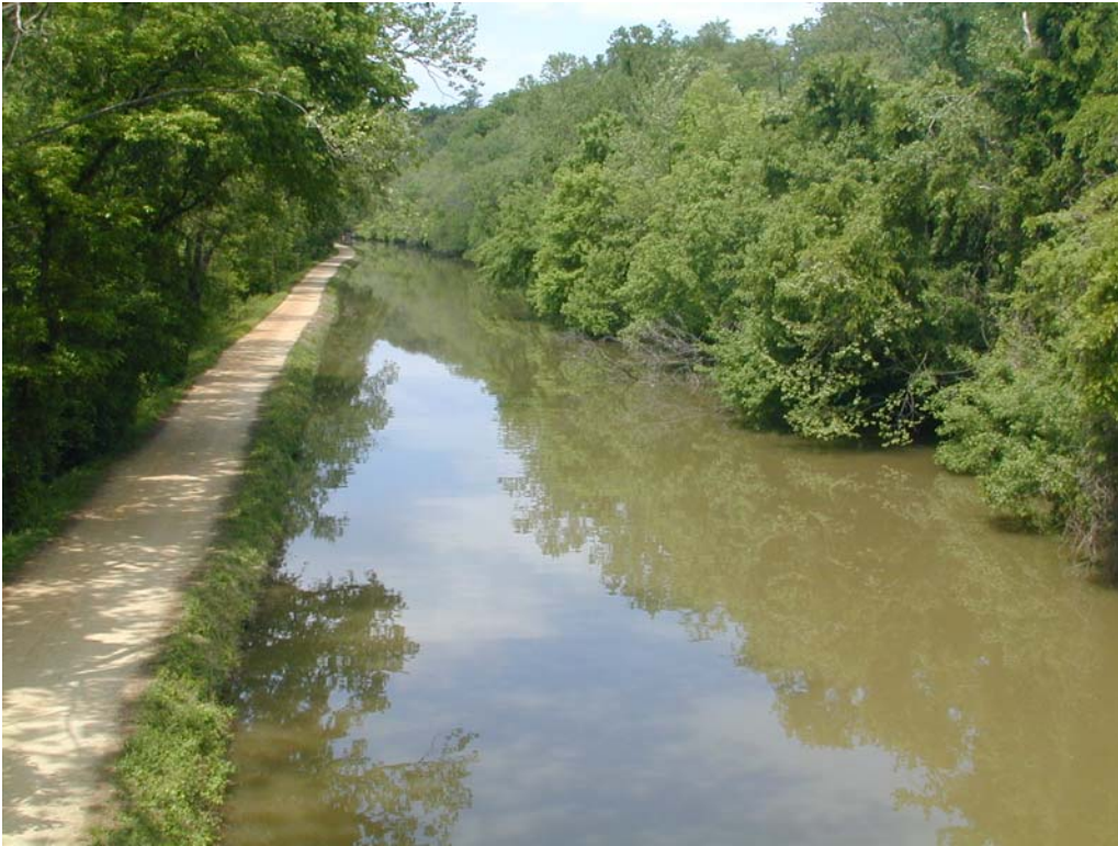
Figure 2-2: C&O Canal at Chain Bridge Road, near District/Maryland Border
