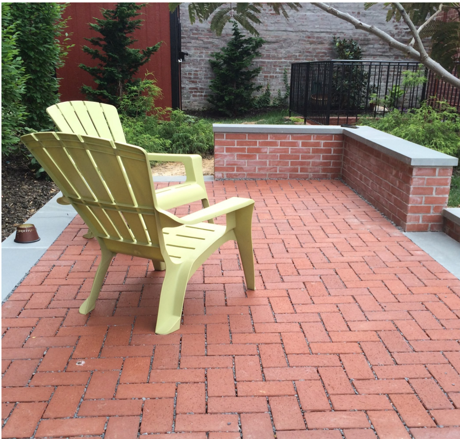
RiverSmart Rebate Pervious Paver Patio
