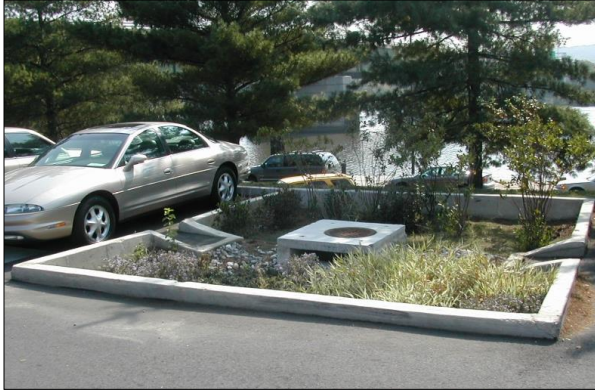
Example of stormwater planter at Navy Yard in SE DC.
