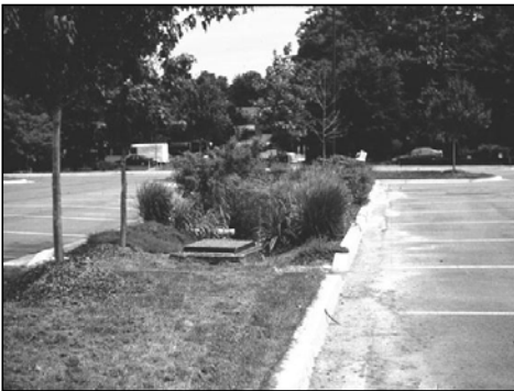
Figure 2: Parking Lot Island Turned Bioretention
