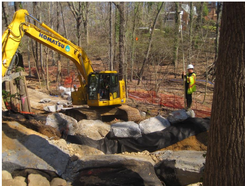
Figure 6: Contractors install stone weir cascade structures from an outfall at Alger Park
