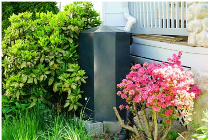
Figure 2: A recently installed RiverSmart Homes rain barrel.
