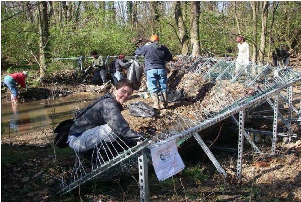
In FY 2009, the District funded the Anacostia Riverkeeper and the Earth Conservation Corps (ECC) to install a Bandalong<sup>®</sup> Litter Trap at the mouth of Watts Branch, a tributary just south of Nash Run (See Figures 7 and 8). This installation marks the first time a device of this type had been installed in the western hemisphere. At the close of FY 2010, ECC estimated that 6,405 lbs of trash and debris were collected by the Bandalong since its installation.
