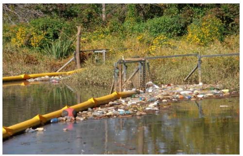
Figure 8 Trash Trap Installed at River Terrace Park MS4 Outfall
