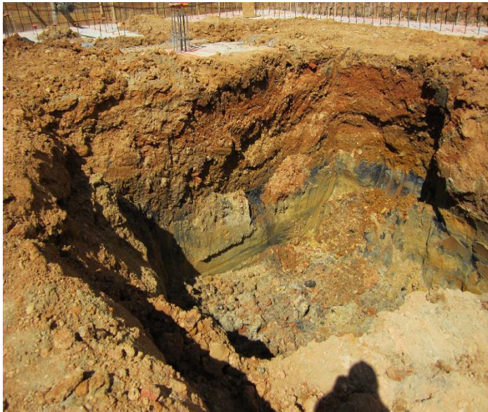
Elevator shaft excavation( stained soil horizon with LNAPL seep )
