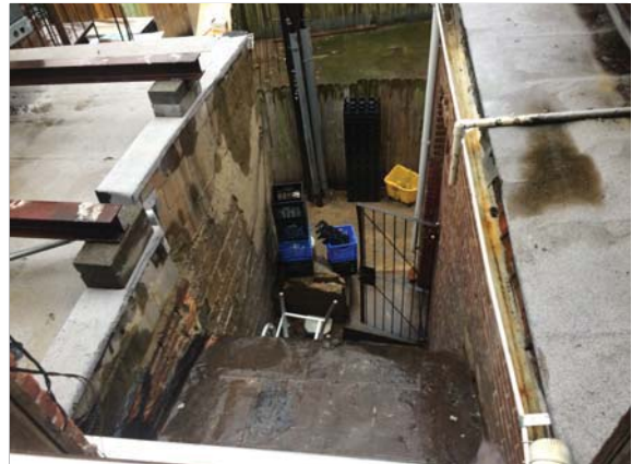
PHOTO 6: Rear alleyway - view from 2nd floor
