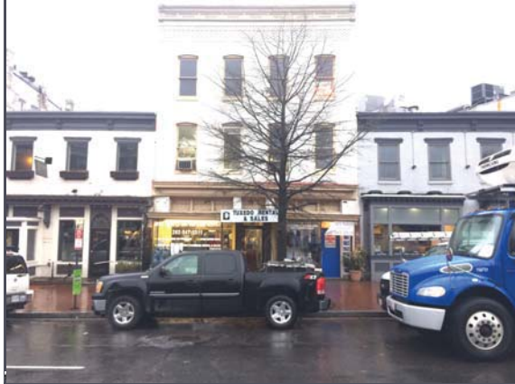
PHOTO 1: Front of building.
