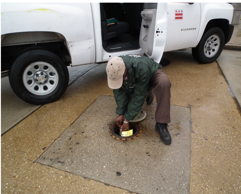
NPS - Brentwood Maintenance Facility, 515 New York Avenue, NE; Tagging 4K gallon diesel UST that was overfilled on Tuesday, May 10, 2016
