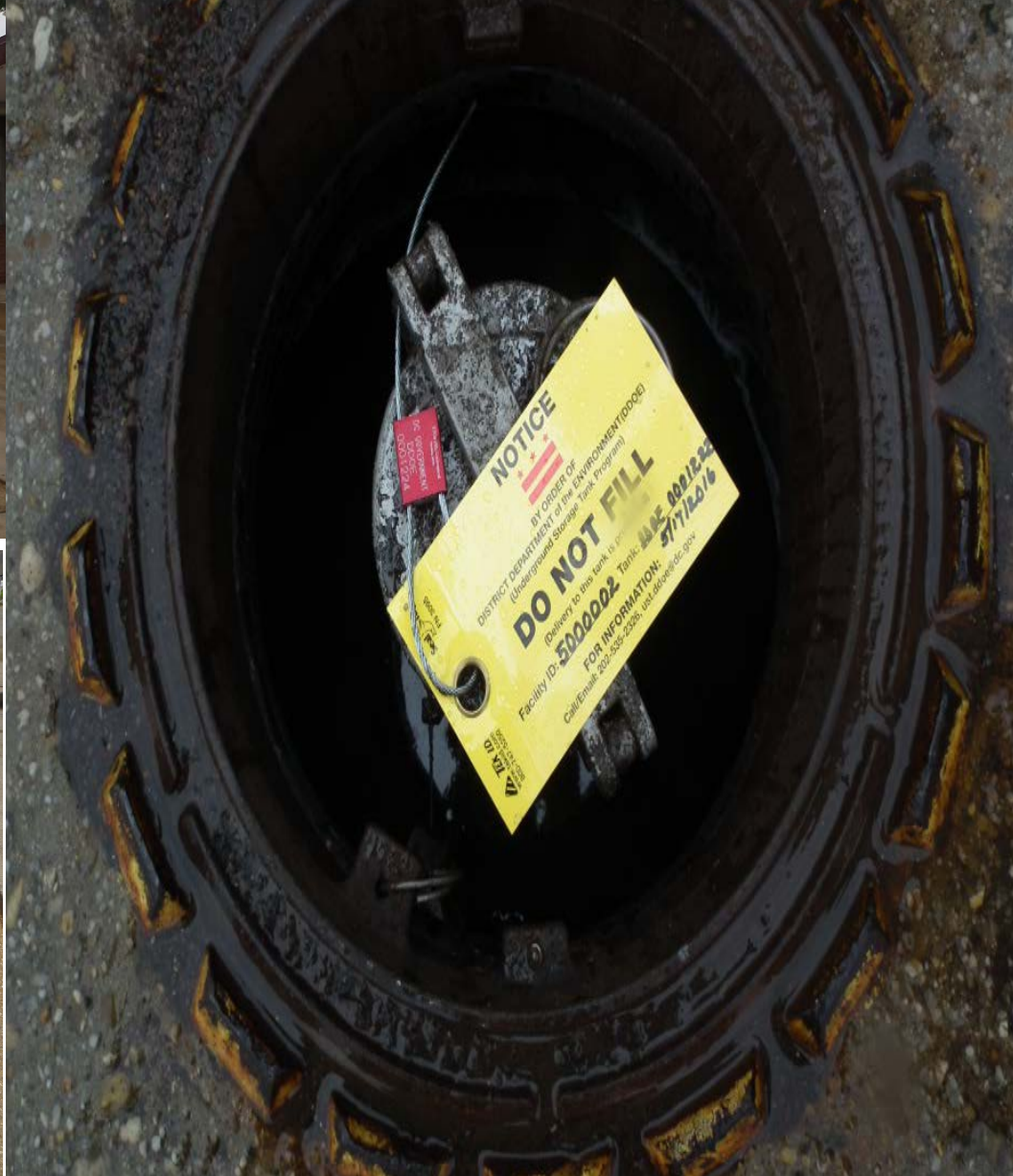
NPS - Brentwood Maintenance Facility, 515 New York Avenue, NE; Tagging 4K gallon diesel UST that was overfilled on Tuesday, May 10, 2016
