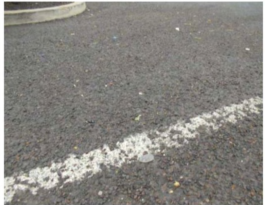
Loose Gravel on Pavement Surface
