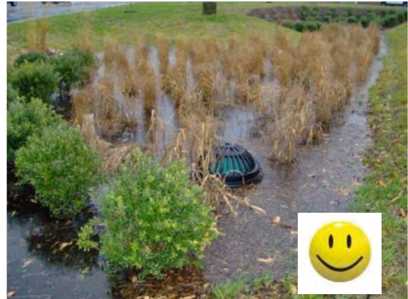
Level filter bed - even distribution of flow across surface
