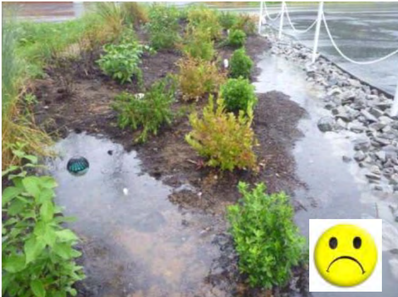
Unlevel filter bed concentrates water in only one area ; uneven filtering
