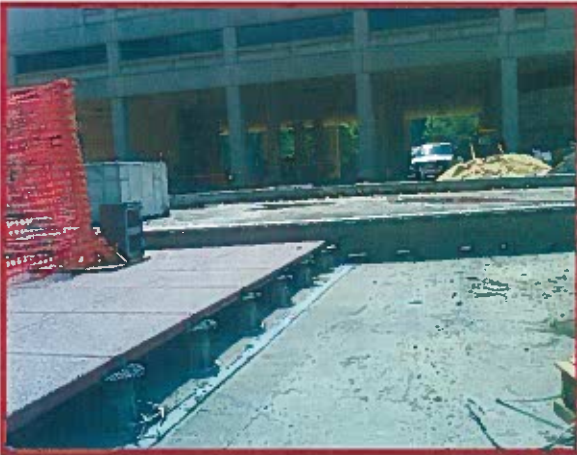
Installation of new cisterns (top left & right) and raised pavers (bottom left) on UDC Van Ness campus for collection of stormwater runoff.
