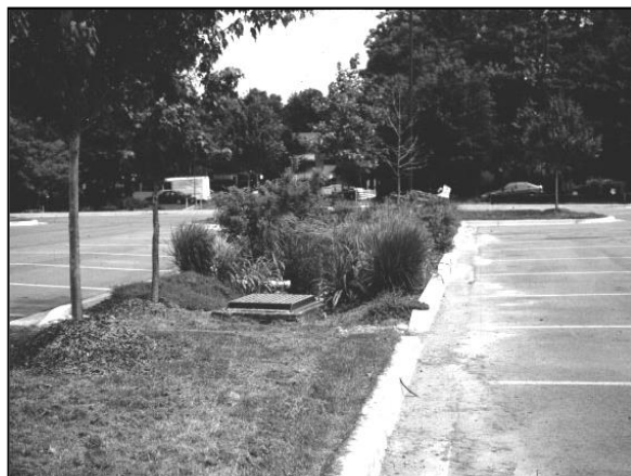
Figure 2: Parking Lot Island Turned Bioretention Area
