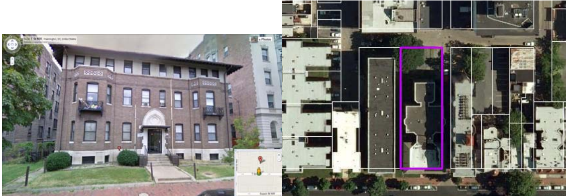
Figure J1. 1433 T Street NW, looking north and aerial, note tree and parking area to the north.
