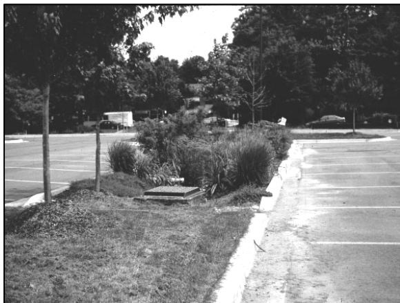
Figure 2: Parking Lot Island Turned Bioretention Area
