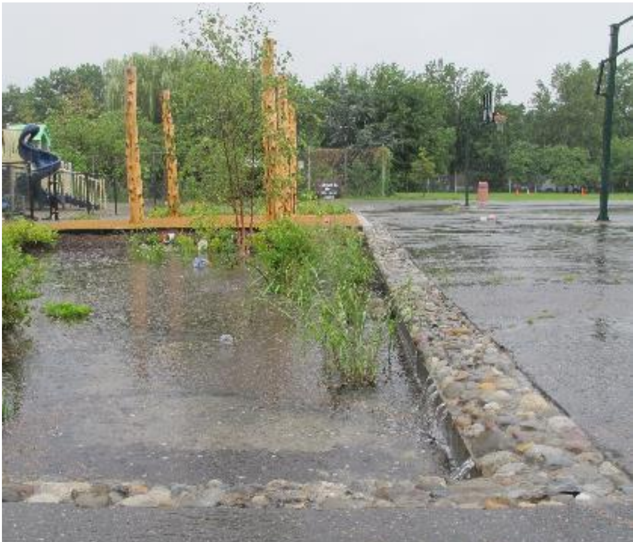
Figure 3: A bioretention project treating stormwater at Seaton Elementary.
