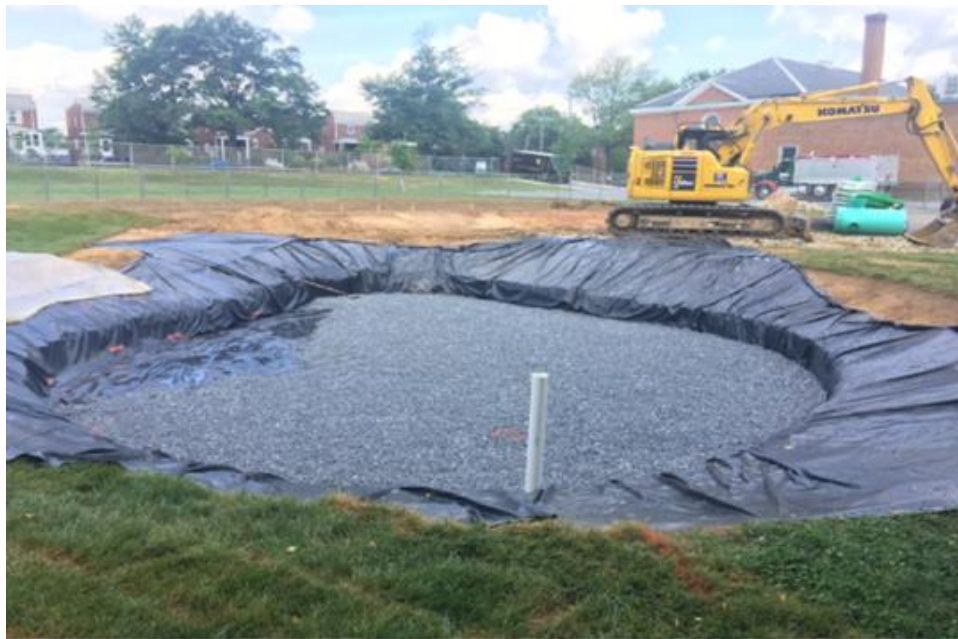
Figure 5: A RiverSmart Schools bioretention basin at Bunker Hill Elementary School
