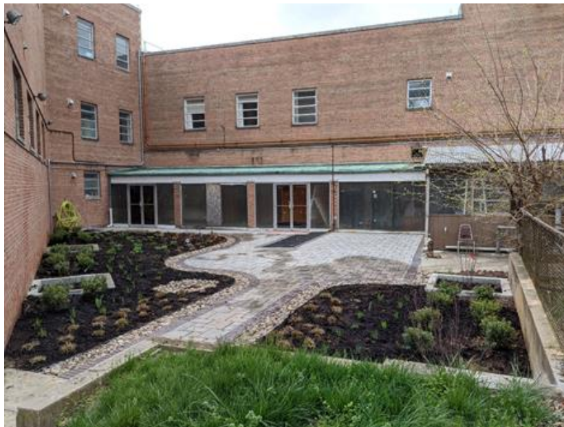
Figure 3: Completed permeable paver installation at Nineteenth Street Baptist Church
