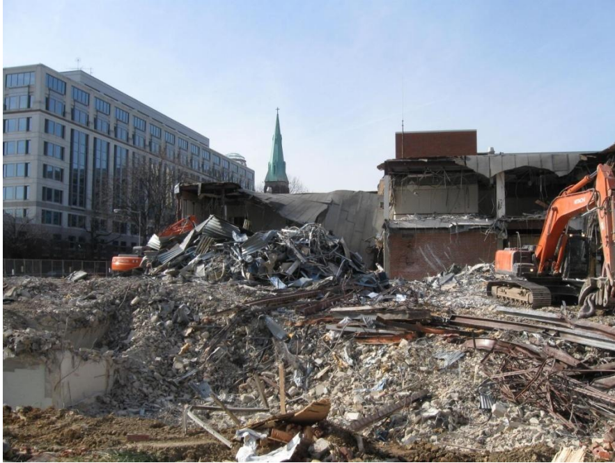
Construction/Demolition First MPD District
