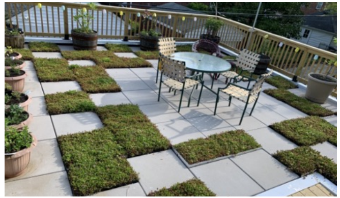
Figure 5: Green roof installation in Ward 4
