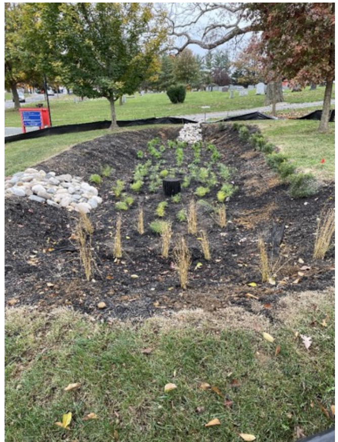
Figure 7: Bioretention installation at St. Paul's Church in Ward 4
