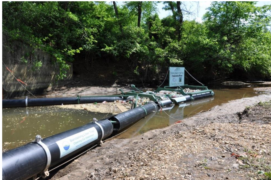
Figure 4: Fund revenues support the maintenance of this trash trap, which removes trash from the Watts Branch tributary of the Anacostia River.
