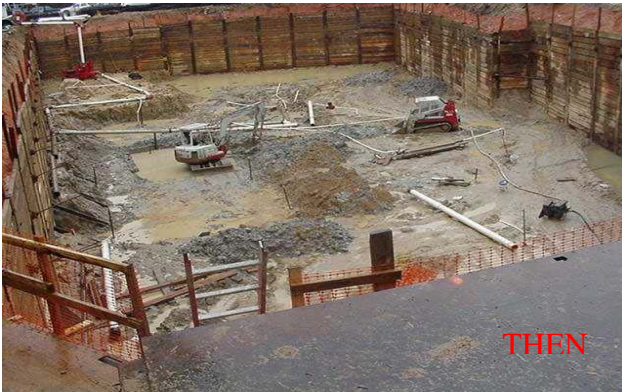
Above – Site under Construction
