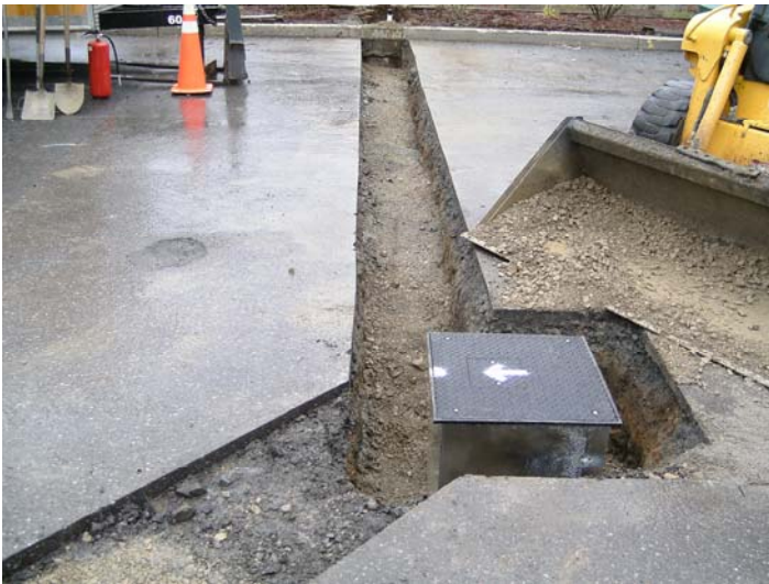
TRENCHING FOR REMEDIATION SYSTEM
