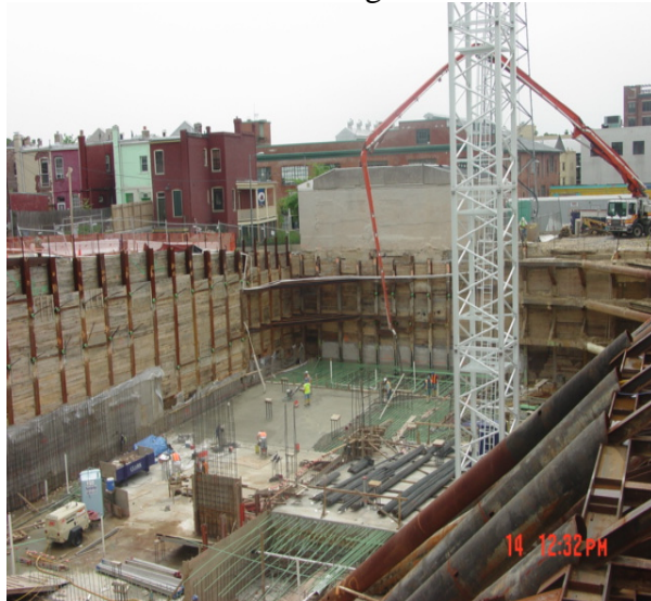
Foundation Work and Tank Removal
