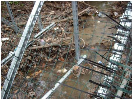
Metal Fence was placed just underneath of the 1"inch mesh plastic net.
