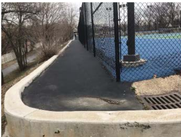
Tennis court curb and inlet
