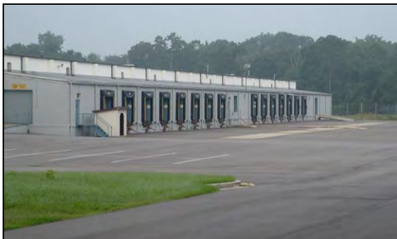
Figure 1: Loading/Unloading Area of Warehouse
