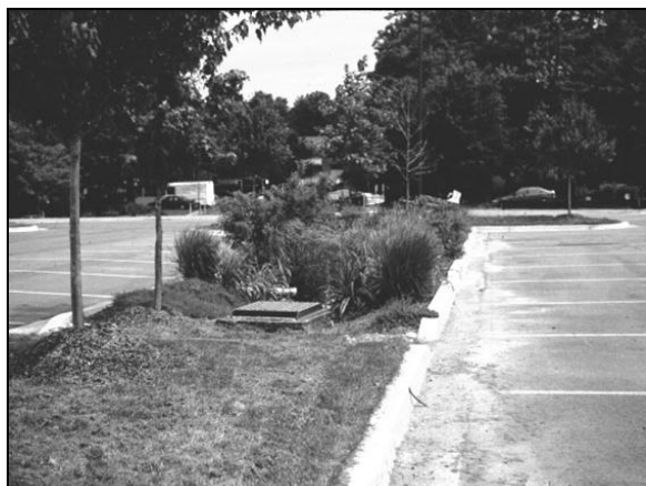
Figure 2: Parking Lot Island Turned Bioretention
