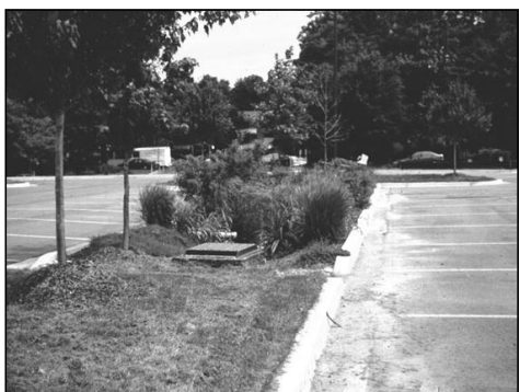
Figure 2: Parking Lot Island Turned Bioretention
