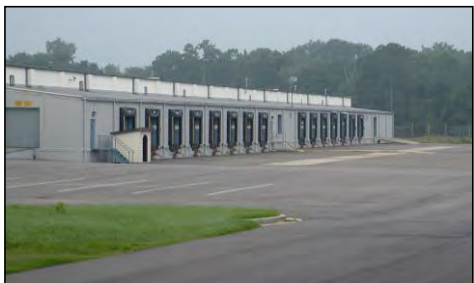
Figure 1: Loading/Unloading Area of Warehouse
