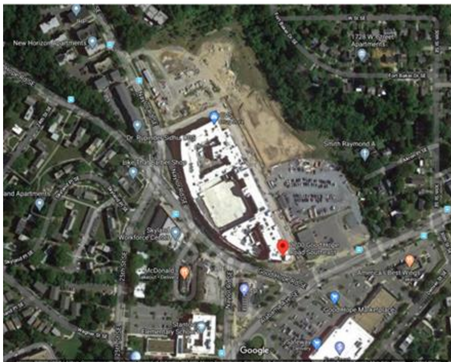
The Skyland Town Center Site is located on Good Hope Road, Southeast DC (Google Satellite Map 2020)
