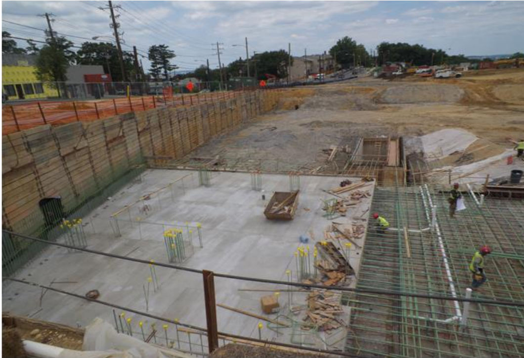
Site during development – showing petroleum vapor barrier under concrete slab -2018
