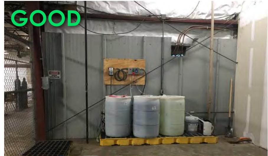
*These supplies are elevated off the ground on pallets & covered with a tarp*
