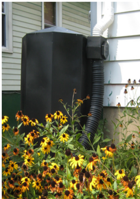
A 132-gallon rain barrel installed at a demonstration site.
