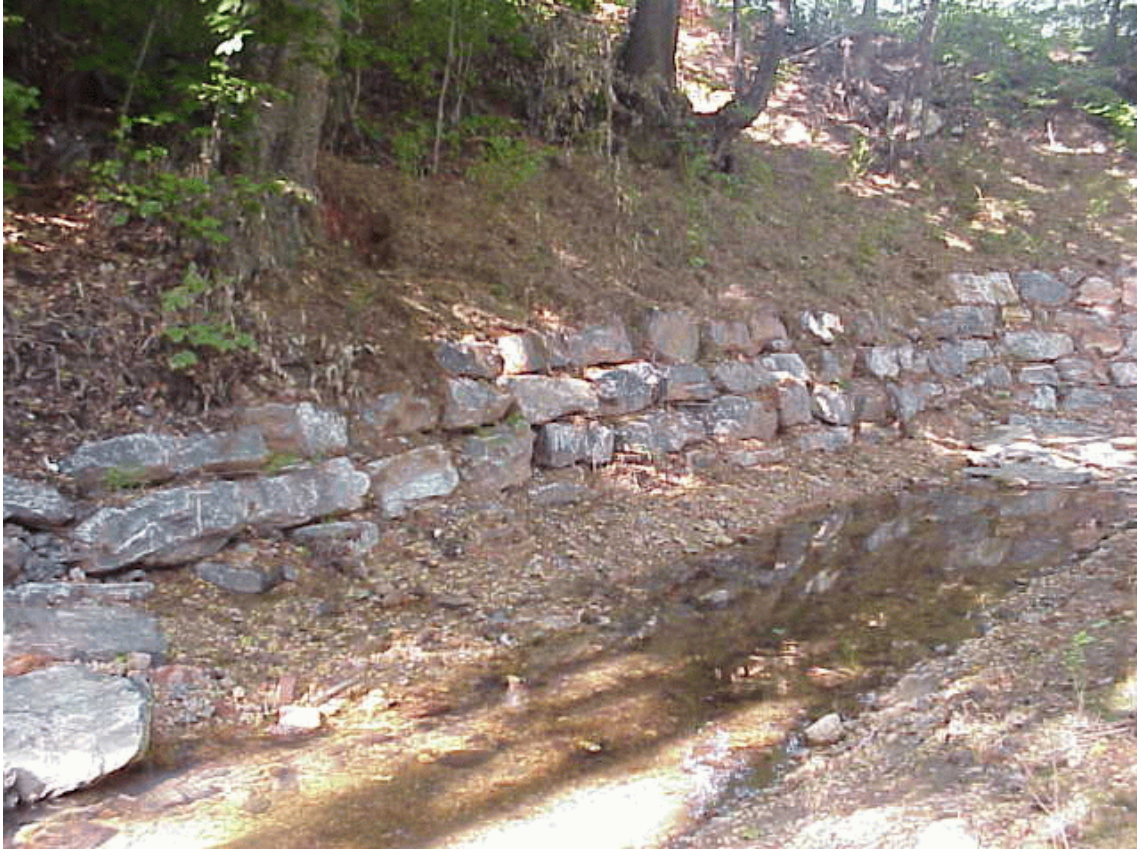
Watts Branch, note the vandal resistant 2 ft. x 3 ft. x 6 ft imbricated rip-rap.
