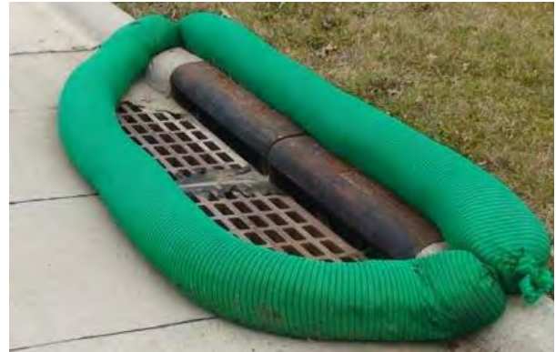
Figure 3.2 Curb inlet protection method
