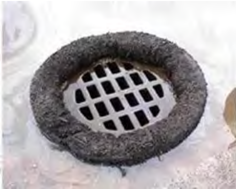
Figure 3.1 At-grade inlet protection method.
