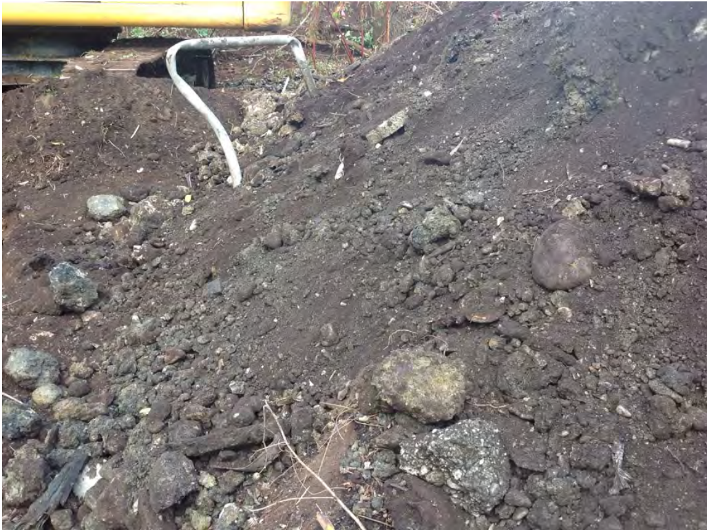
Photo 5: Excavated material consists of construction debris mixed with organic soil.
