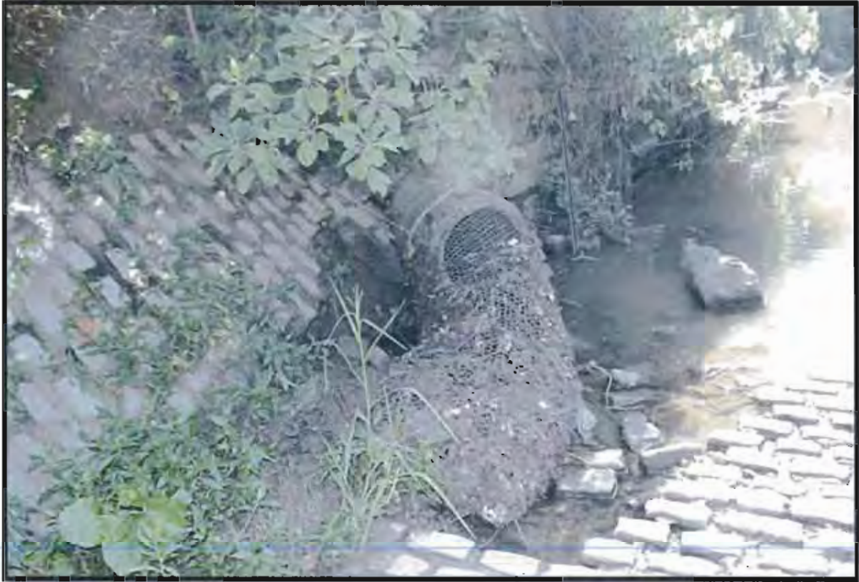
Figure 3 Sock style trash trap at McDonald's Outfall. Socks for monitoring will be longer to allow more room for water to escape before hitting the trash accumulating at the toe.
