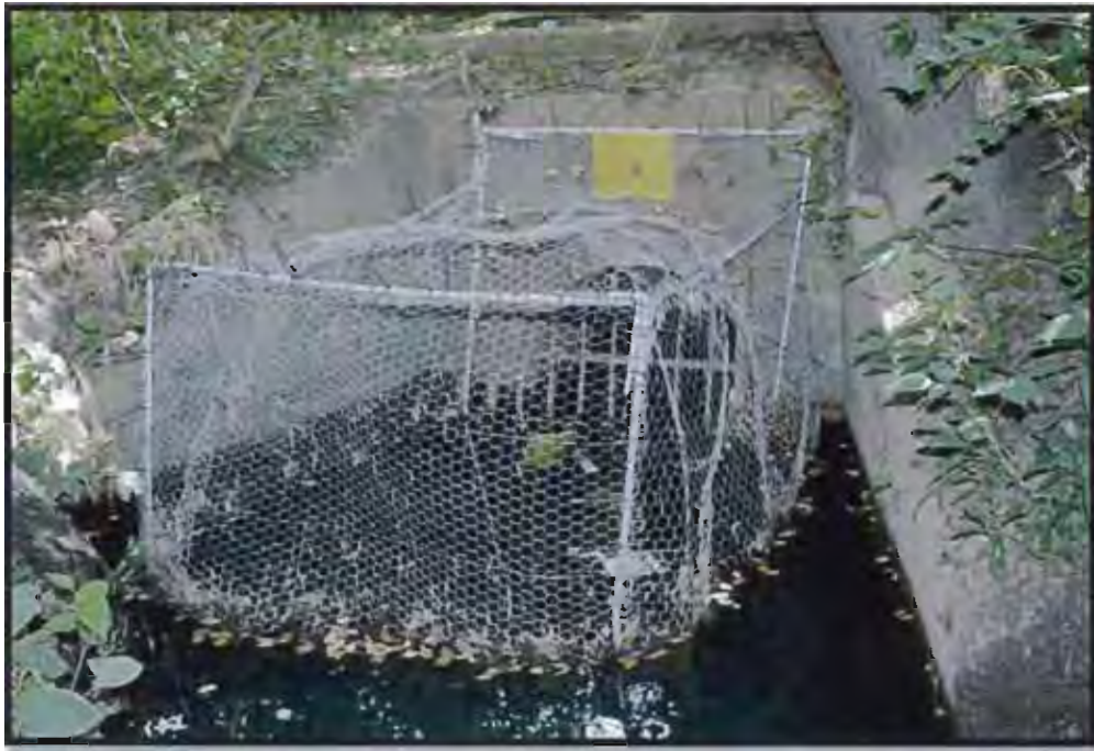
Figure 2 Box Trash Trap on Meade Outfall.
