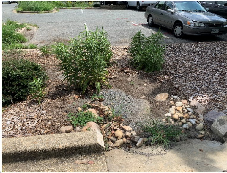
Figure 1. Example of sediment and debris accumulation in bioretention inlet
