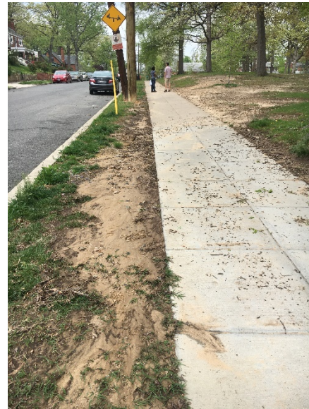
Figure 2 (left): Example of compacted ‘pervious’ space in the District; Figure 3 (right): Sediment runoff into public right-of-way from compacted open space in District.
