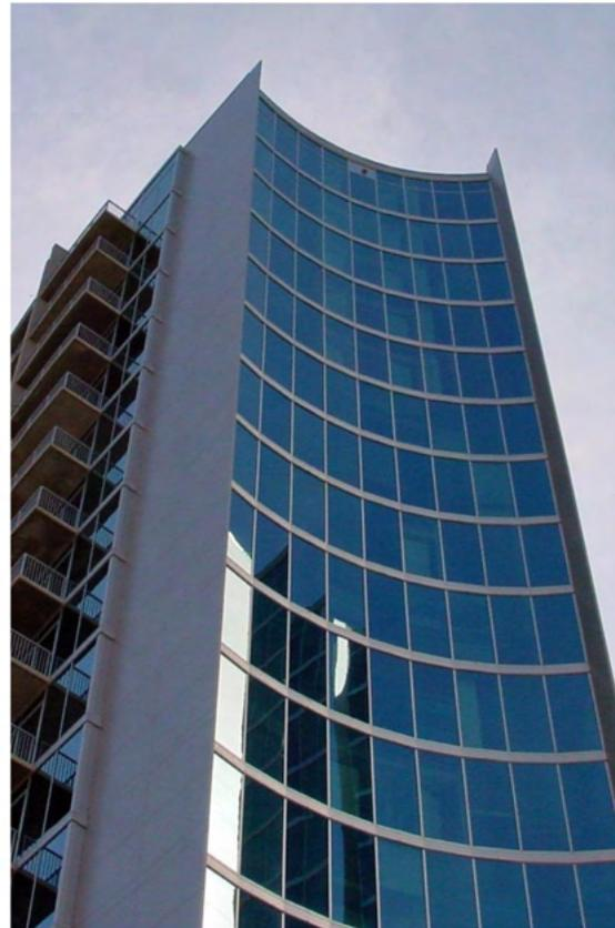
Window wall systems are commonly used in ribbon window configurations or punched openings as shown here on the Plaza Midtown building in Atlanta, GA.
