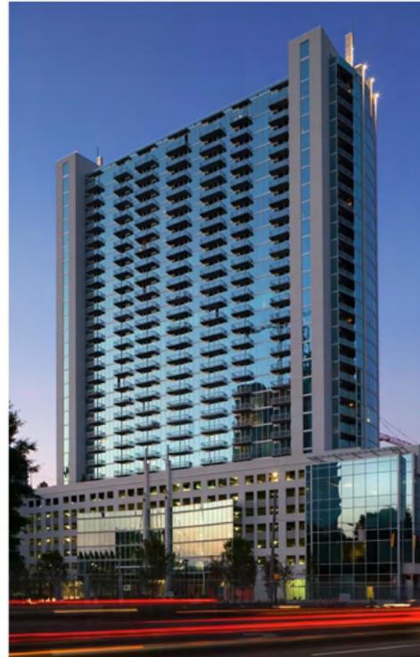
Window Wall offers the look of a true curtain wall with a slab-to-slab aluminum frame design with a slab edge cover option to conceal the floor slab. Kawneer products are comprised of extrusions made from one of the earth's most plentiful recyclables — aluminum. Durable and lasting the extruded products also boast aesthetically appealing design features that can help contribute to energy efficiency and long term sustainability.
