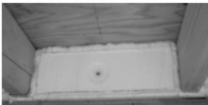
Don't use fiberglass batts to insulate between rim joists because air can move around the fiberglass, causing condensation and encouraging mold on the cold rim joist. If you use foam to insulate between the rim joists, use liquid foam sealant to seal around the edges of the rigid foam.
