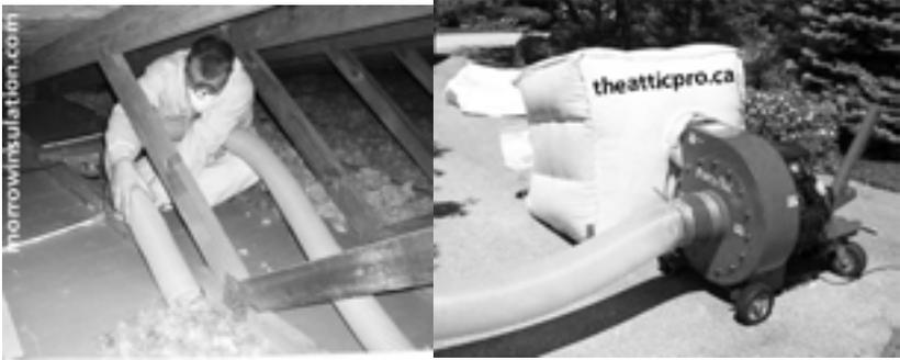
**Removing attic insulation:** Technicians vacuum and collect existing attic insulation for re-use or disposal because of moisture damage or to allow effective air sealing.
