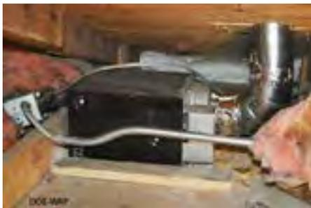
**Right-way fan orientation:** Air stream turns 90 degrees which is acceptable.
