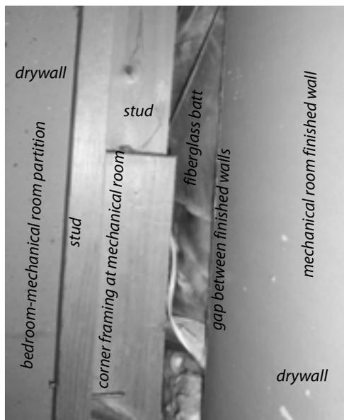
**Large air leak in finished basement walls:** Two finished basement walls meet inside a mechanical room and form a 2-inch gap from floor to ceiling connecting the finished basement with the space behind its finished walls.
