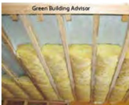
**Flash and batt:** An inch of high-pressure foam seals the cavities and the correctly-sized batts complete the insulation job.
