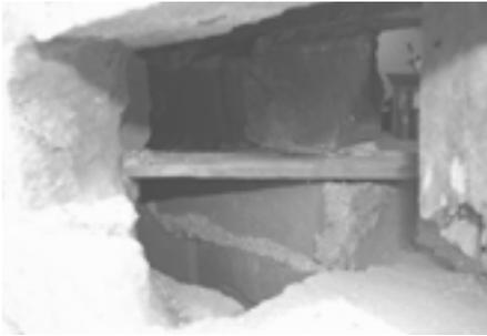
**Cavity brick wall:** Two separate single brick walls are held together by wood lath embedded in the mortar joint.
