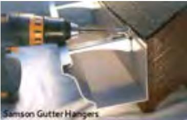
**Gutter hangers:** Reinforced gutter hangers prevent snow and ice from detaching gutters from the building.
