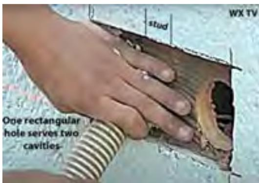
**One hole fills two cavities:** Use a pattern to mark the rectangular hole.
