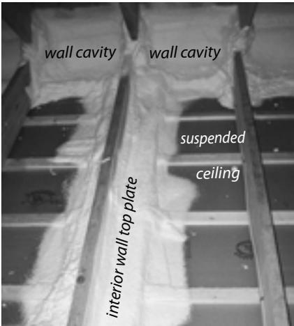
**Sealing structural suspended ceilings:** Two-part foam air seals and insulates an interior wall top plate and the wall cavity between the ceiling and roof deck.
