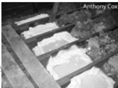
**Kitchen soffits:** The ventilated attic is connected to the soffit and the wall cavity through framing flaws. Any hole in the soffit creates a direct connection between the kitchen and attic. Block off the soffit from the attic with drywall or plywood sealed with two-part spray foam as shown in the photo.
