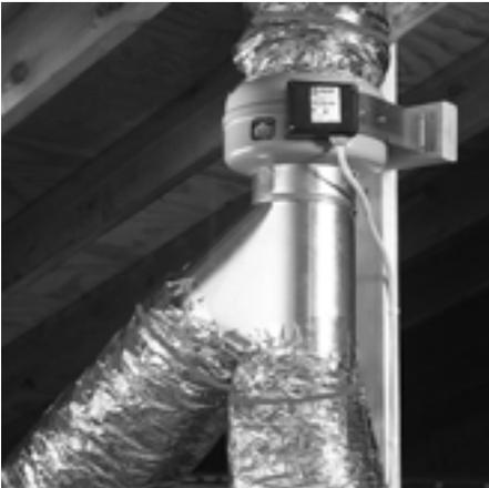
**In-line fan in attic:** A Y exhausts airflow from two bathrooms for both local exhaust and whole-building ventilation.
