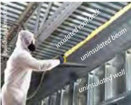
**Sealing the roof deck:** Seal the roof wall junction with spray foam. Insulate the walls above the suspended ceiling. Insulate the roof deck if there's no insulation on top of the roof deck.
