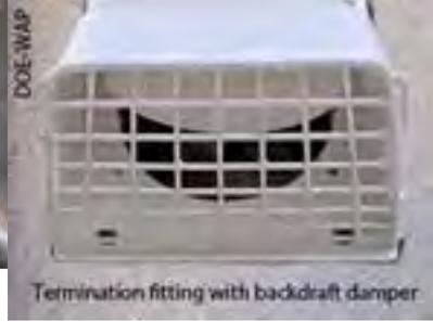
**Vent and termination:** Use rigid metal vent pipe if at all possible. Or use flexible metal vent and not foil vent when flexibility is required.
