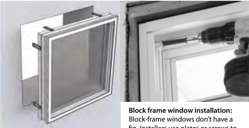
**Block frame window installation:** Block-frame windows don't have a fin. Installers use plates or screws to fasten the window to its opening.
