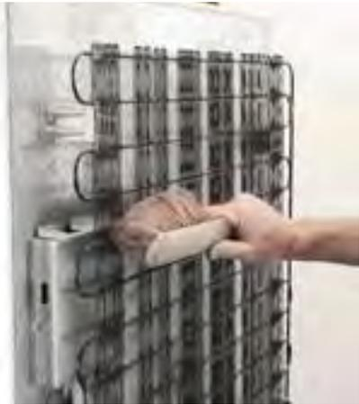
**Refrigerator clean and tune:** Clean coils and check temperatures. Adjust temperatures that are out of range.
