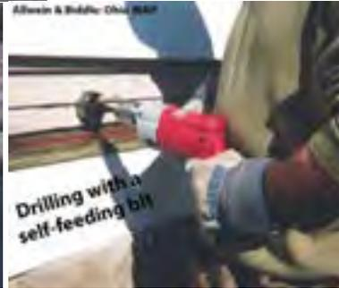
**Remove the lower piece:** Then drill holes for the insulation.
