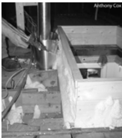
**Two-part foam:** A contractor air-seals and insulates around an attic hatch dam with two-part spray foam.
