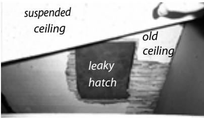
**Sealing existing upper ceilings:** With a non-structural suspended ceiling and a damaged plaster ceiling above, seal the plaster ceiling above if it's impractical to air seal the suspended ceiling.
