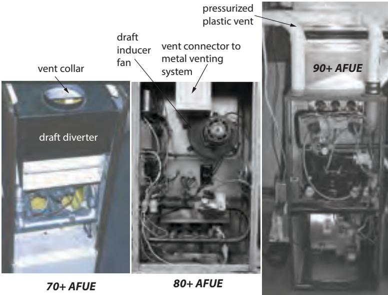
**Gas furnace evolution:** Energy auditors should be able to identify the 3 types of gas and propane furnaces. Only the 90+ AFUE furnace has a pressurized vent. The two earlier models vent into traditional natural-draft chimneys.
