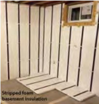
**Installing stripped foam:** Installers glue and screw the foam sheets to the masonry wall and concrete slab. Then they glue drywall to the foam and screw the drywall to the strips.
