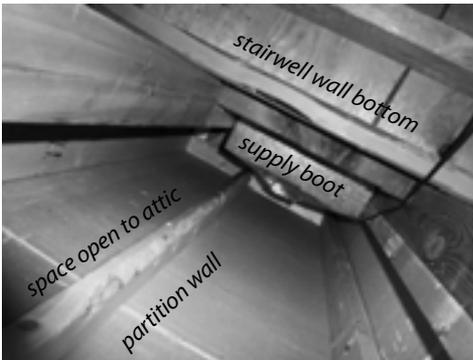
**Stairway wall within the thermal boundary:** Double wall forming the stairwell connects an unfinished area under the basement stairs with the living spaces, attic, and the space behind the finished basement walls.
