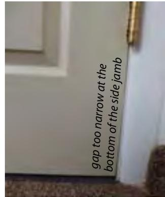
**Symptoms of a sagging door:** Gravity rotated this door to pinch the top jamb side corner and bottom hinge side corner of the door against the side jambs.
