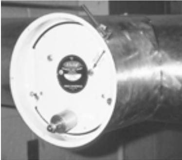
**Barometric draft control:** This control provides a stable overfire draft and controlled flow of combustion gases through the heat exchanger.
