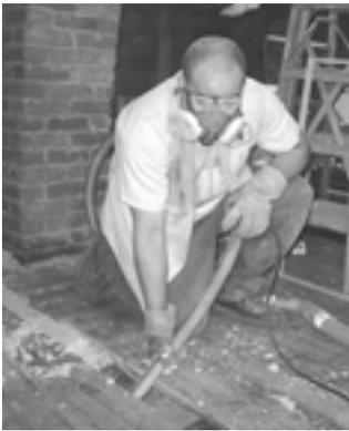
**Finished attic floor:** Find the large air leaks underneath the flooring and seal them before insulating the space between the joists.
