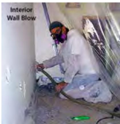
**Tube-filling walls:** perform this method indoors or outdoors. Tube-filling is the preferred wall-insulation method because it achieves a uniform coverage and density.
