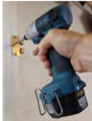
**Solutions for door sagging:** Bend the hinge knuckles slightly, drive a long screw into the hinge, and/or drive another long screw into the jamb above the hinge. Experience will tell you which solution works in each particular case.
