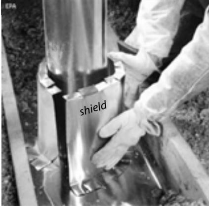
**Sealing manufactured chimneys:** When installing retrofit insulation in addition to air sealing, install a shield on top of the air seal that extends above the level of the new insulation.
