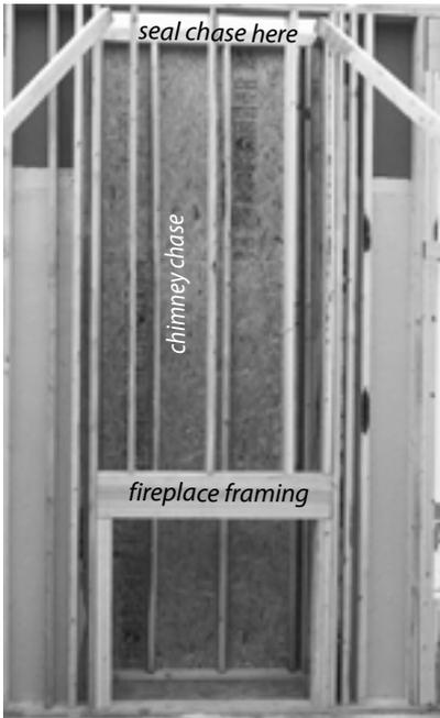
**Chimney chase:** Chimney chases can be multistory air-leak conduits if they're not sealed at floors and ceilings.
