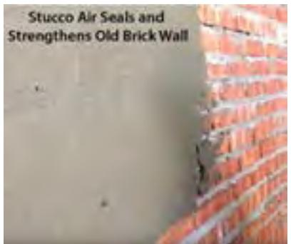
**Stucco over brick:** This retrofit serves two purposes: air sealing and structural reinforcement.
