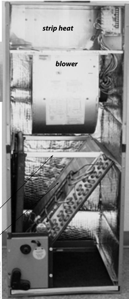
**Heat pump:** This upflow indoor air handler contains a blower, indoor coil, strip heat, and filter bracket.
