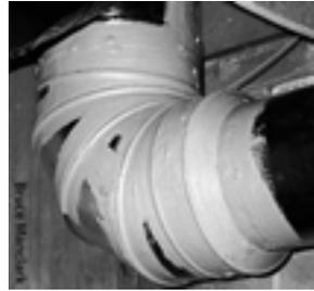
**Plenums, poorly sealed to air handler:** When air handlers are installed in tight spaces, plenums may be poorly fastened and sealed. Cutting a hole in the duct may be the only way to seal this important joint.
