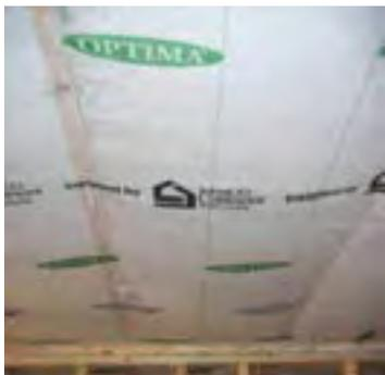
**Insulation restraint:** Workers patched access holes after they blew this floor through an air barrier.
