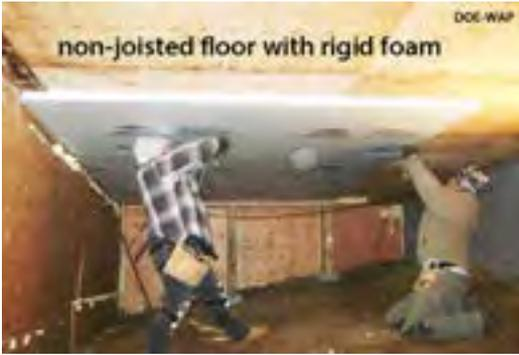
**Non-joisted floors with rigid foam:** Workers fasten rigid foam to a non-joisted floor with plastic-cap nails.
