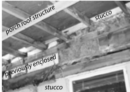
**Porch air leakage:** Porch roof cavities often allow substantial air leakage because of numerous joints, and because there may be no siding or sheathing installed in the wall behind the roof and ceiling.
