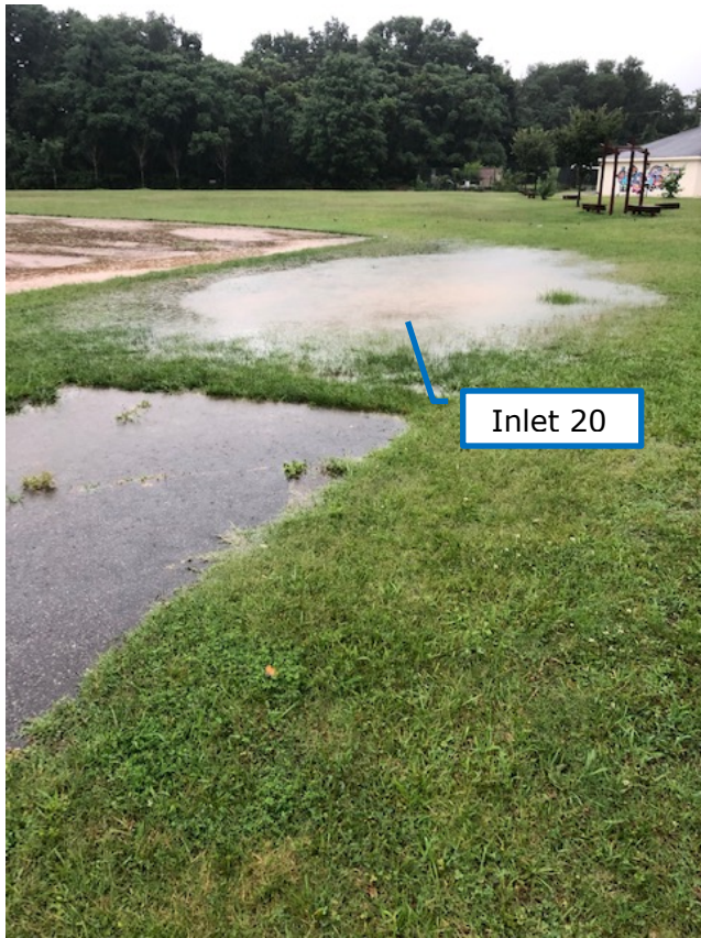
Photo 2- Ponding at Inlet 20
