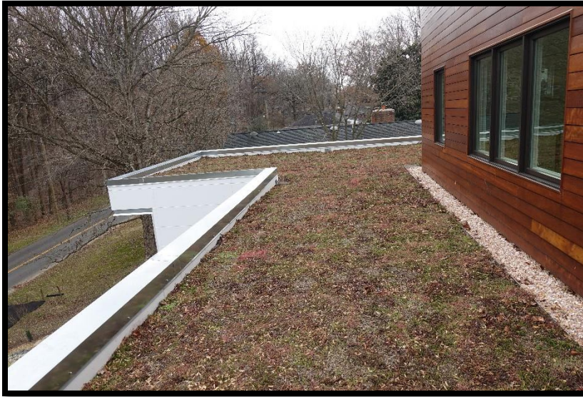
Figure 8 - New Green Roof Installed Through the RiverSmart Rooftops Program in FY 2020
