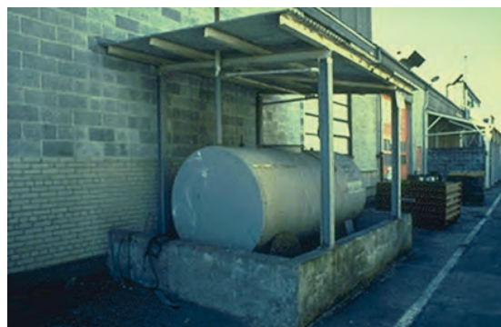
Roof over a diked AST
