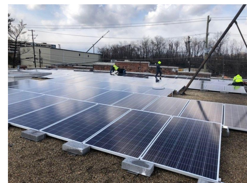
Installation of the solar panels on the roof of AYT Auto Services in Northeast (Photo by Global Consulting, Inc. 2019)
