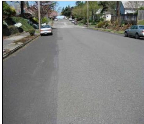
Installation of permeable, or porous asphalt in the parking lanes and conventional asphalt in the drive lanes in Portland, OR.
