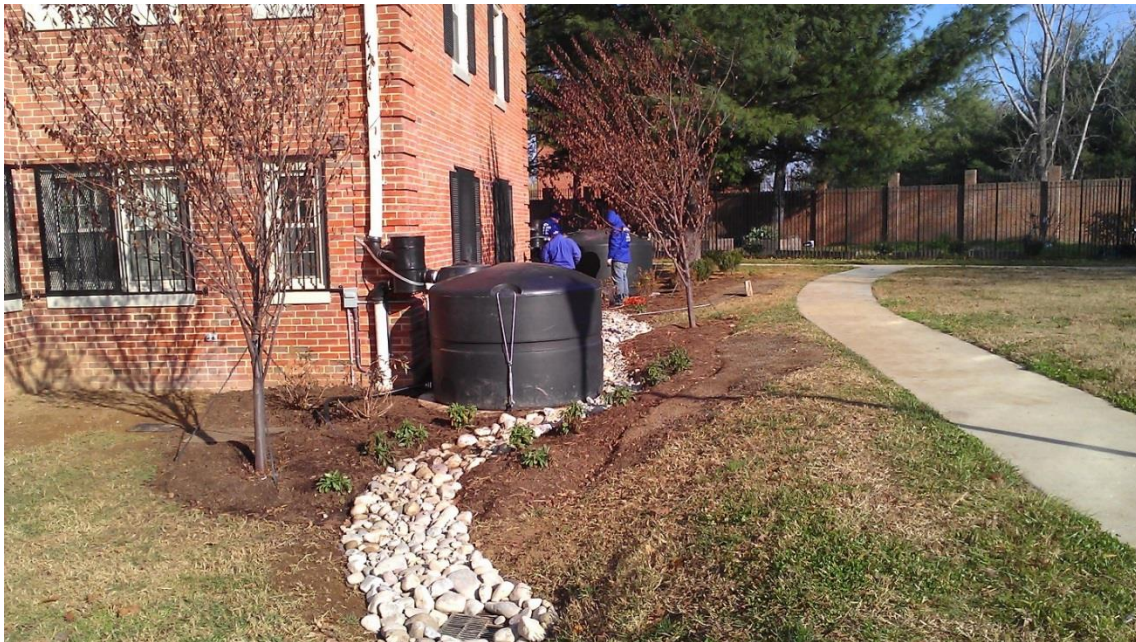
Example of a large cistern to capture roof runoff and supply water to the garden (Mayfair Mansions)
