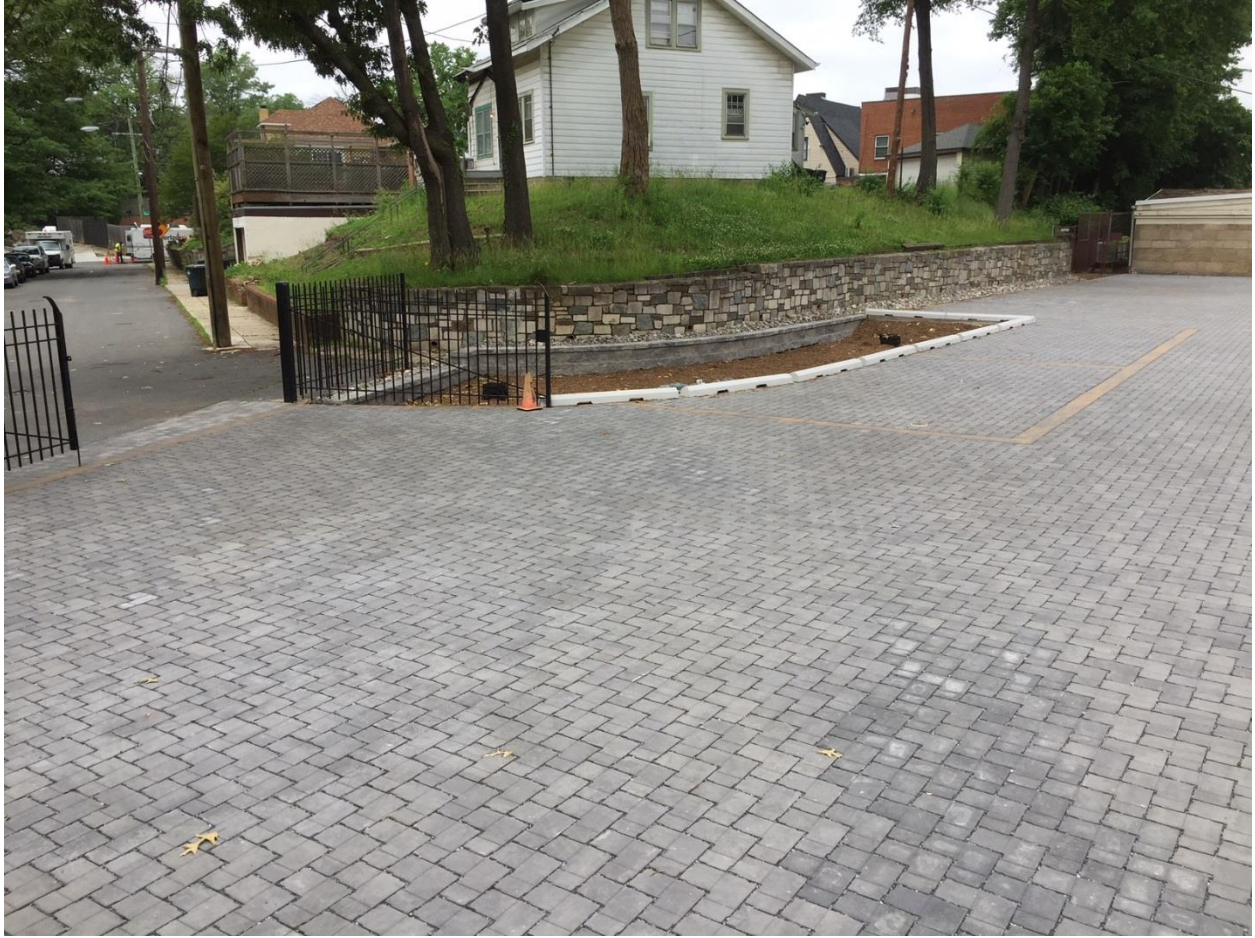
Example of pervious pavement parking lot at St. Francis de Sales in Ward 5.
