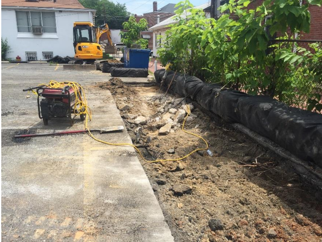
Example of impervious surface (asphalt) removal from the parking lot of Morningstar Baptist Church.
