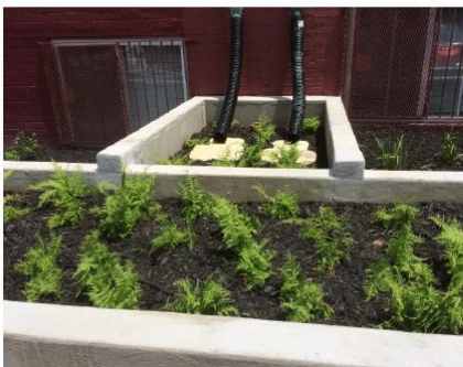
Example of stormwater planter installation (Galen Terrace).
