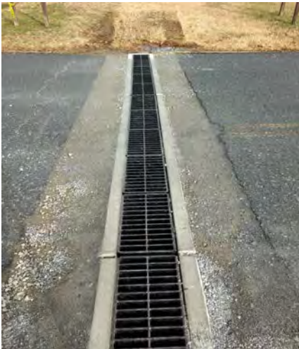
Photos 4 and 5: Trench Drain
