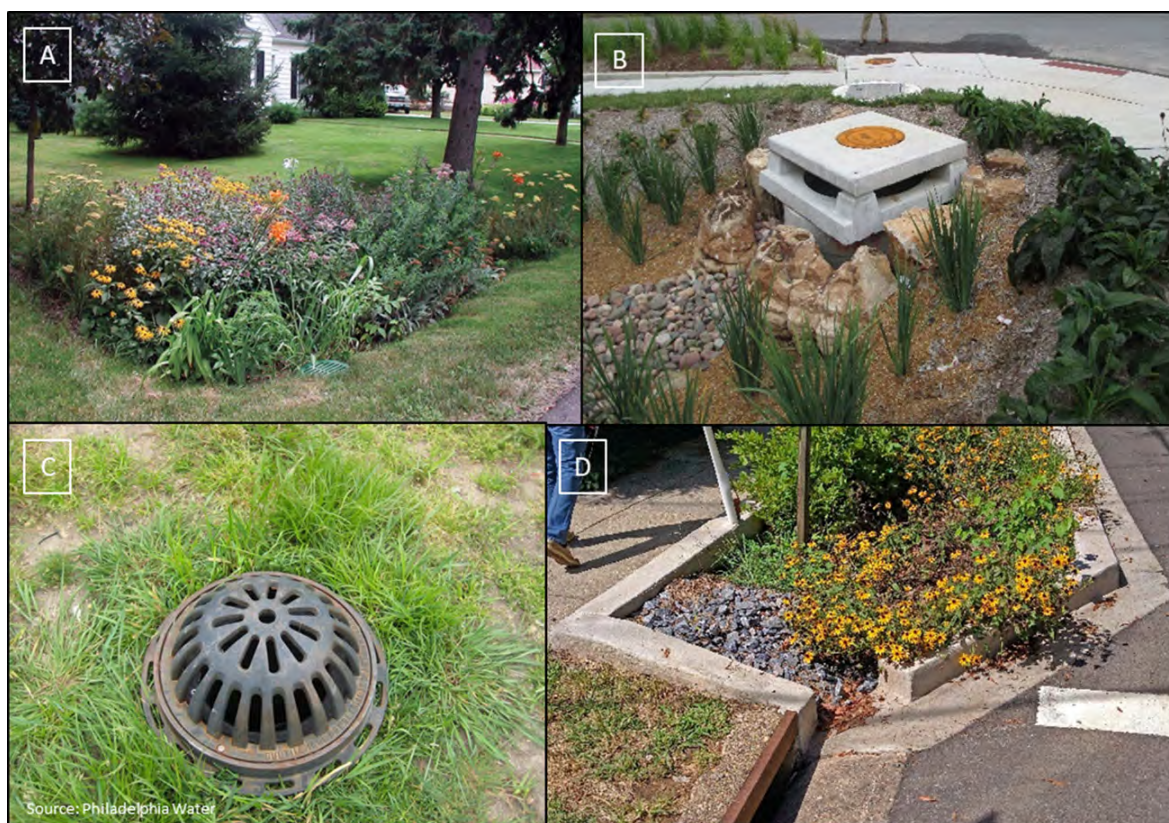
Figure 13: (A) Vegetation in bioretention. (B) and (C) Overflow structures. (D) Curb cut for runoff to flow into bioretention
