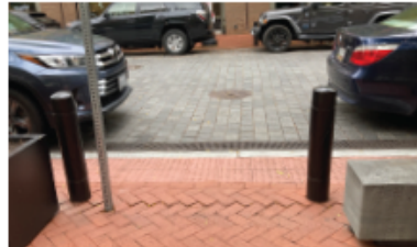
"Tabled Streets" at Eastern Market, DC using flush curbs, trench drains, and Permeable Pavement (Top Left, Top Right)
